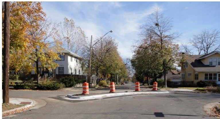
Figure 6.9 – Diagonal road closure
