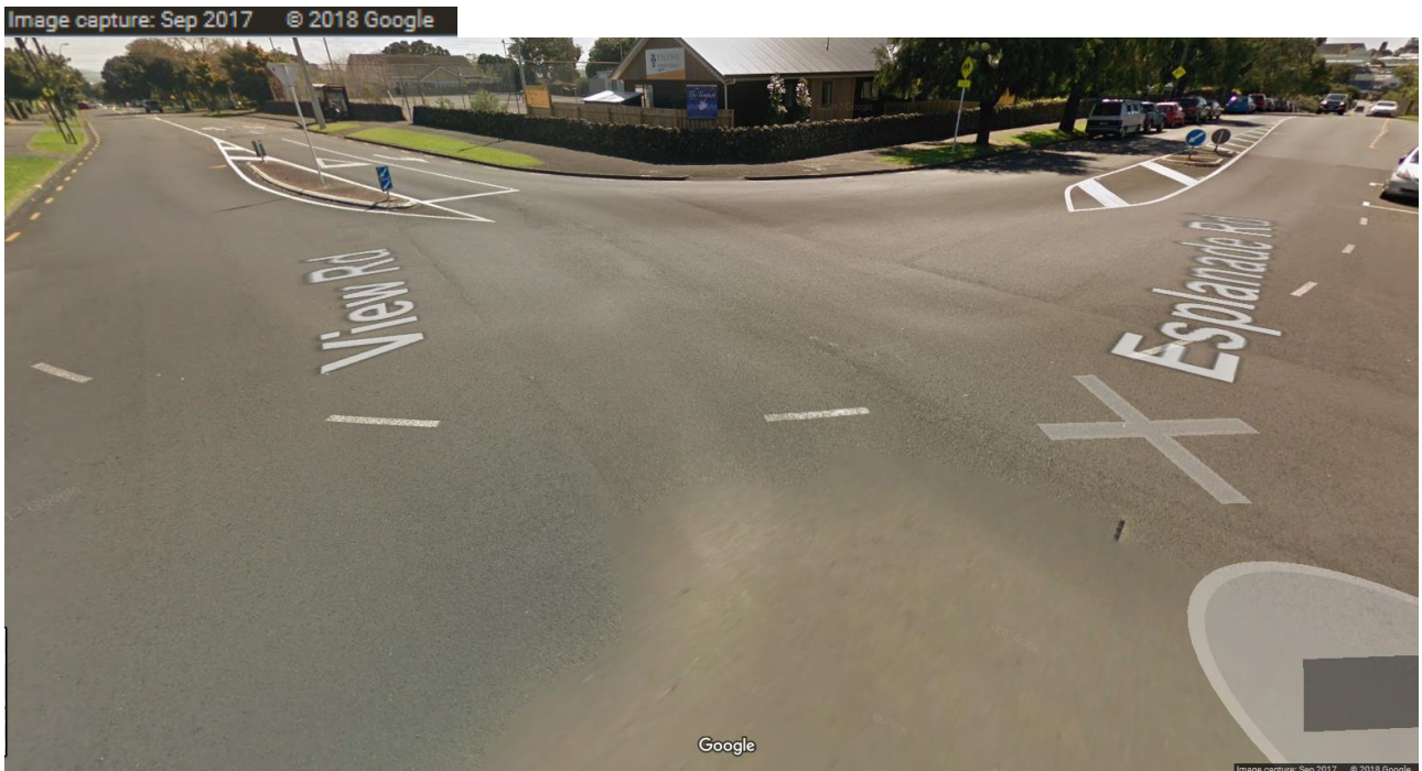
Figure 6.6 – Modified priority intersection
