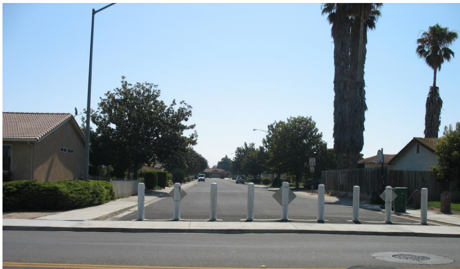
Figure 6.11– Full road closure
